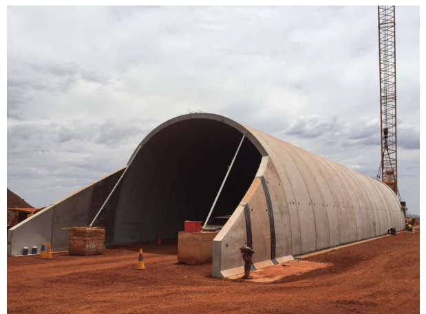
RIO TINTO'S , HOPE DOWNS HV TUNNEL WA - NPI
