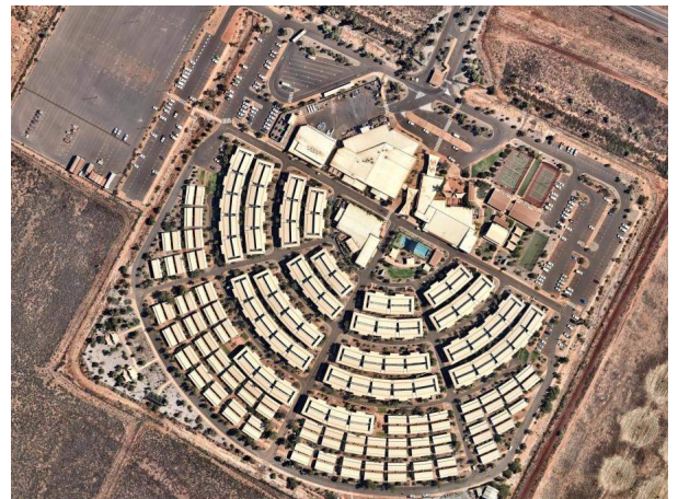
BHP'S PORT HAVEN CENTRAL FACILITIES - NPI
